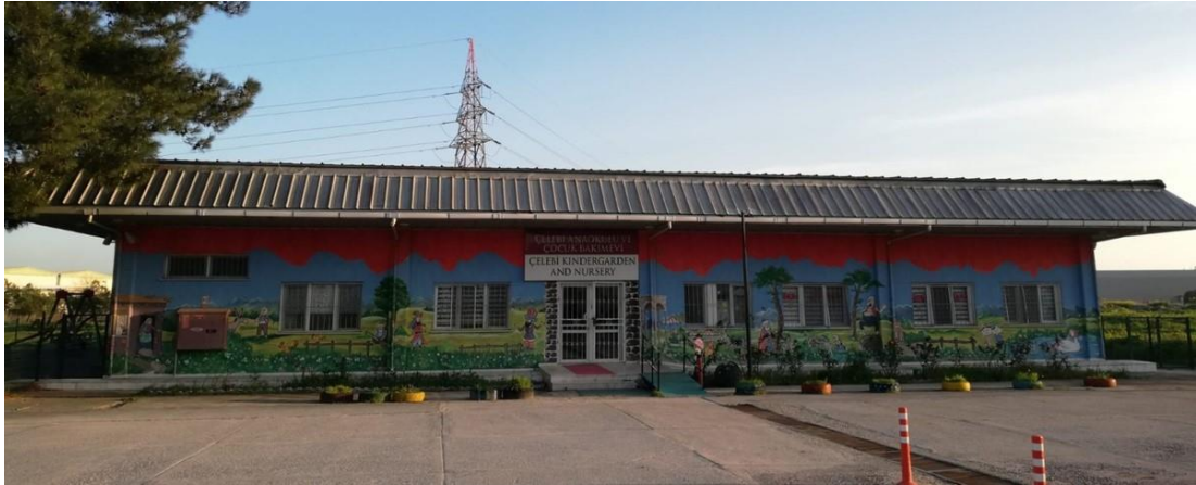
Figure 2.1: IKCU daycare building (front view)
